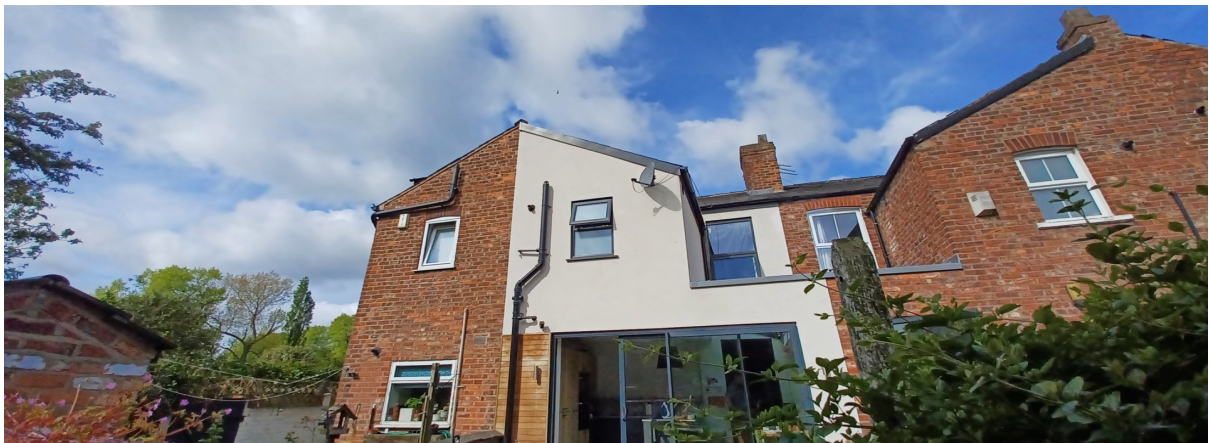
Figure 6. Rear roof of property.
