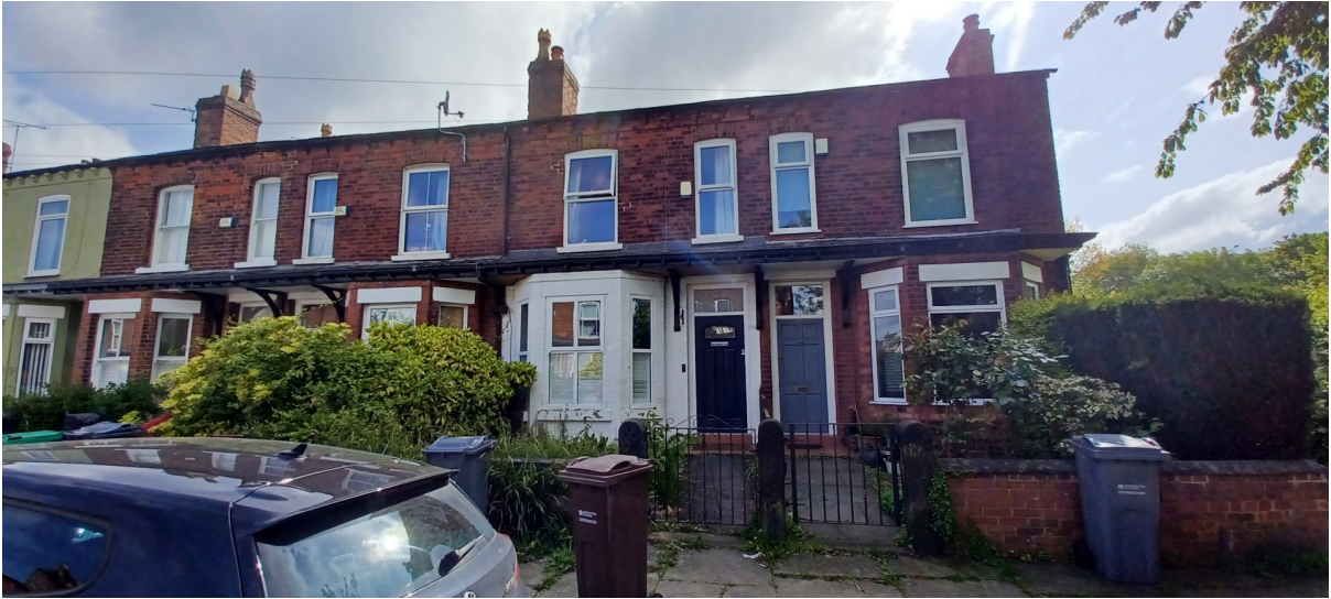
Figure 3. Principal elevation of property.
